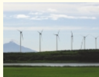
Wind power generators at Teshio River in Hokkaido.
